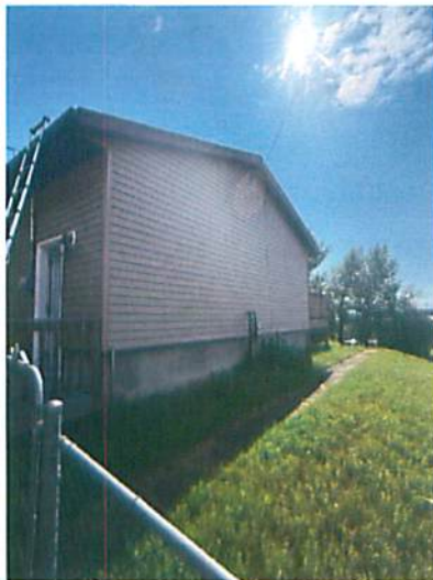
Photograph of exterior vinyl siding and Cementous parging. June23, 2026
