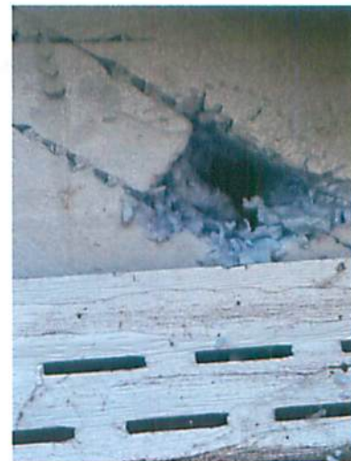
Photograph of Styrofoam insulation between sheathing and vinyl siding. Insulation section was removed to assess for possible ACM stucco exterior however only Tyvek paper on sheathing found. June23, 2026
