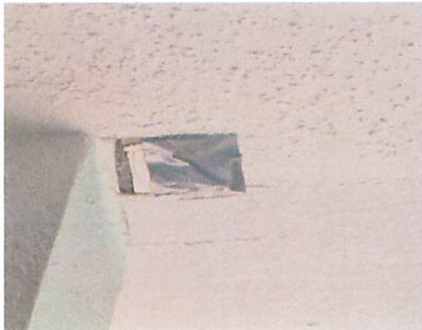
Ceiling Texture in Basement
