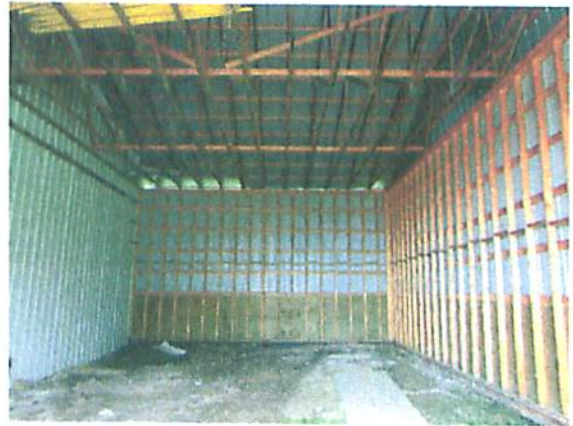
Interior of Attached Shelter
